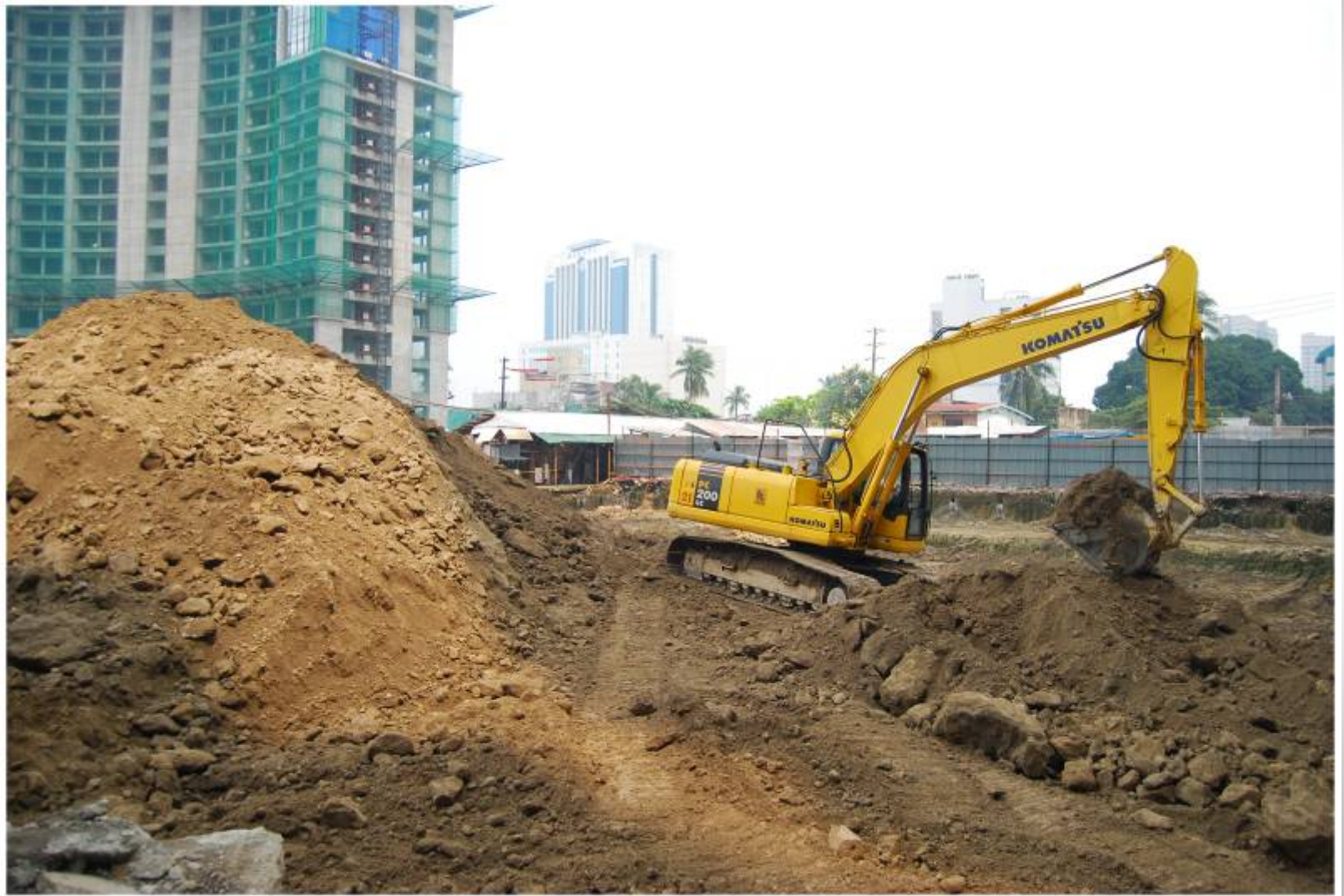
A photo of Centuria's construction site with excavation works in progress
