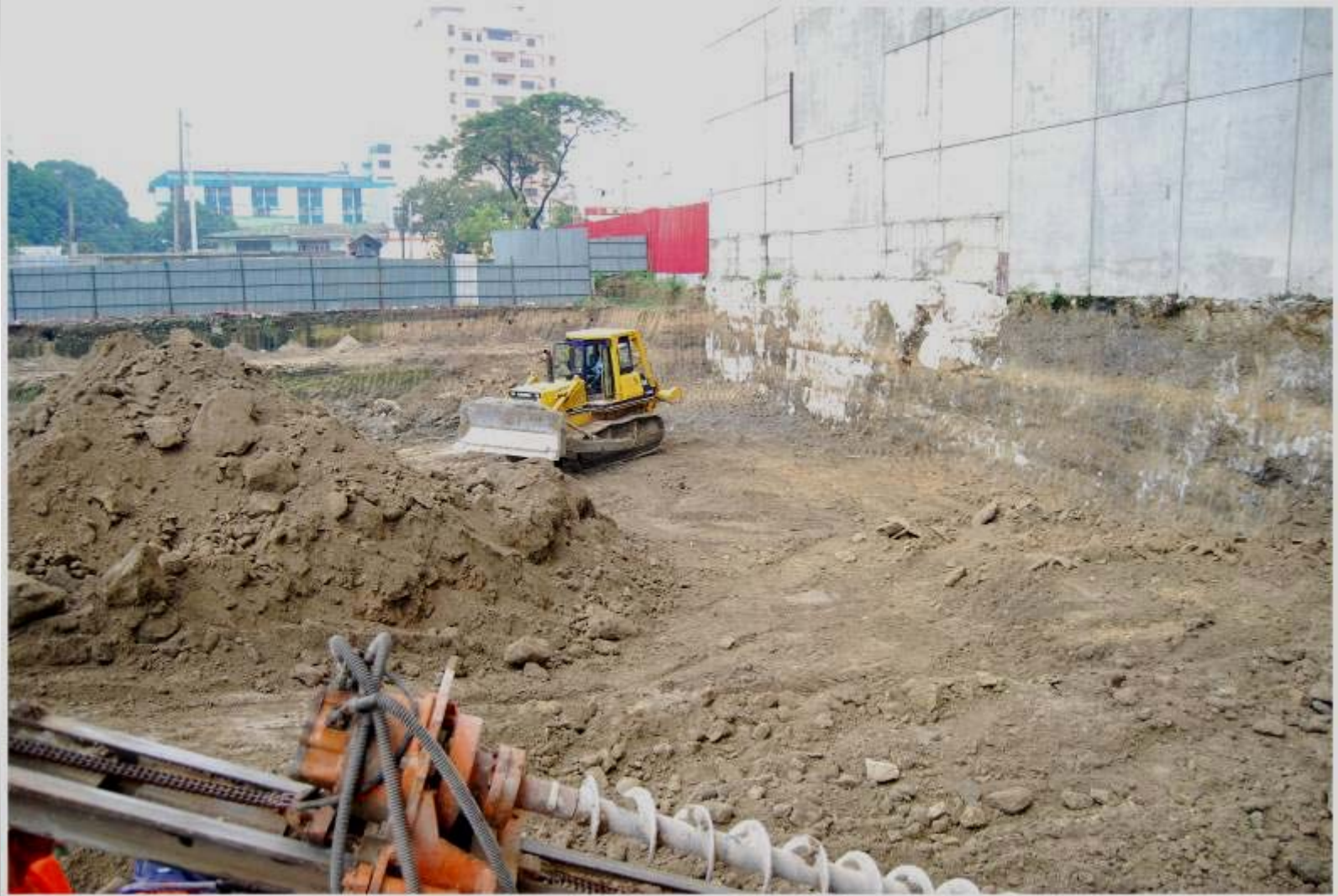
Another photo of the excavation works at the Centuria site
